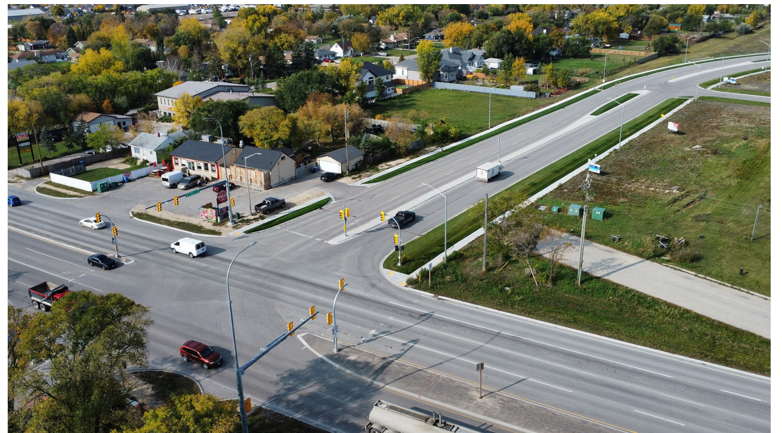
Main Street and Meadowlands Drive controlled intersection
